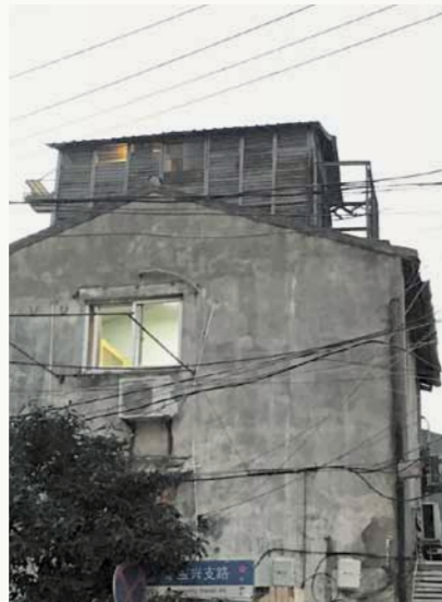
A self-built incremental attic might be used as a studio or bedroom despite considerations about street facades and structural safety (Jin Zhu)
