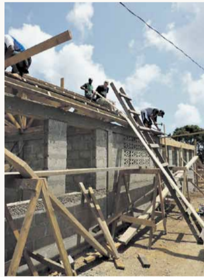
Constructing a hazard-resistant school in Puerto Cabezas (Eefje Hendriks)
