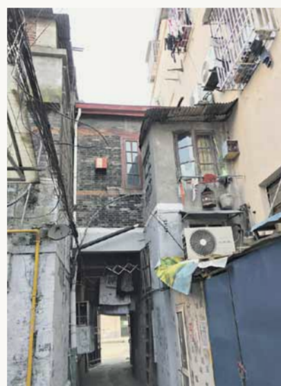
In a narrow lane, an incremental two-storey structure “grows” parasitically beside the facade of Old Communal Housing (Jin Zhu)
