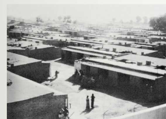
Community centre / View of a typical unit (ASAG / Kirtee Shah)
